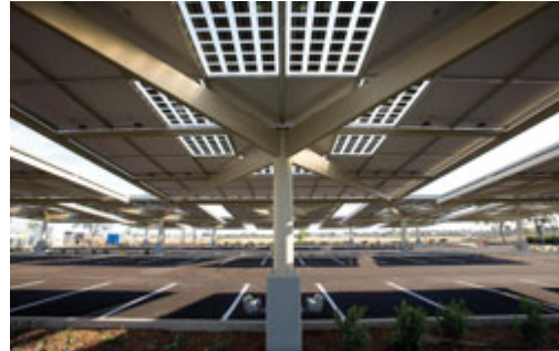
The Solar Tree parking system can store and generate solar energy.
