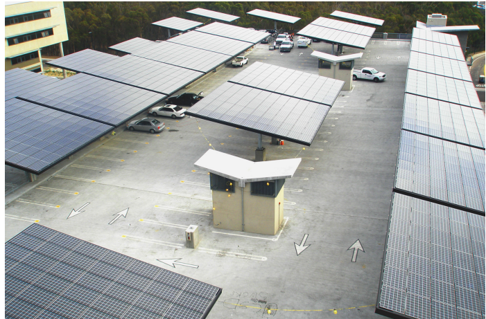
University of California San Diego Hopkins Parking Structure
