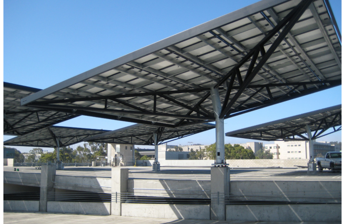
University of California San Diego Gilman Parking Structure
