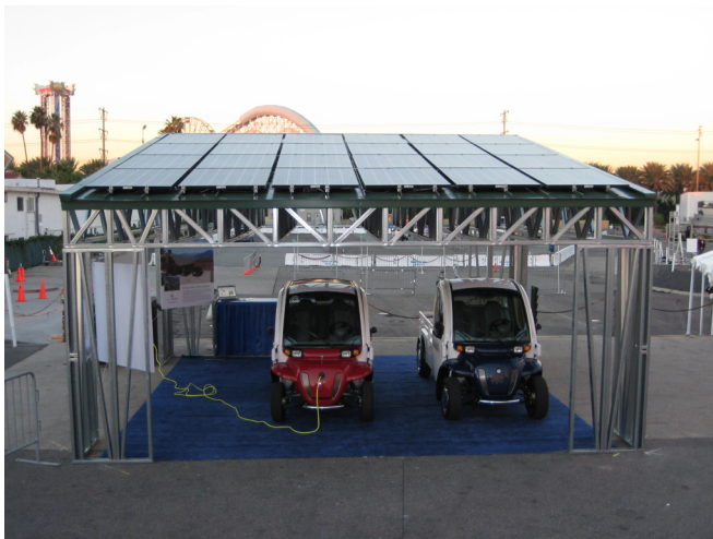
Envision Solar displays its LifePort solar structure, generating energy to power two electric vehicles.
