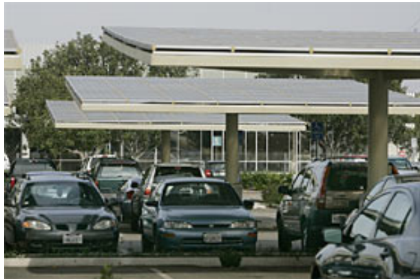
JOHN GIBBONS | Union Tribune At the Kyocera facility, parking areas are covered by “solar trees.” There are obstacles for solar parking arrays, including the rising cost of steel needed to build them.
